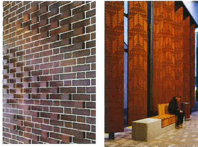
Timber panel and bespoke brick pattern at entrance to be developed through cultural narrative process
